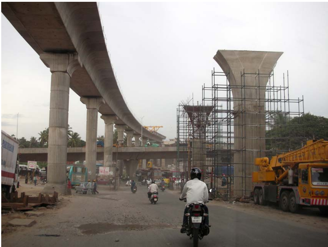
Road and metro construction in Bangalore, 2012
