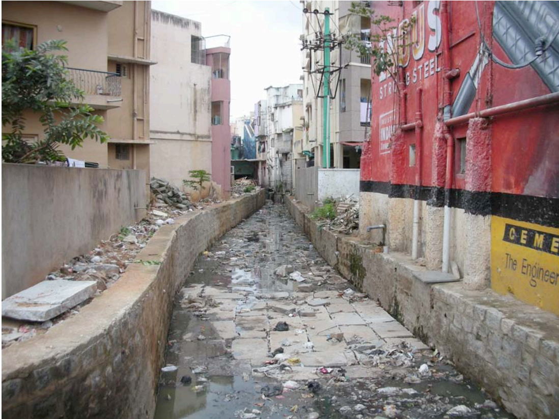
Storm-water drain in Bangalore, 2012
