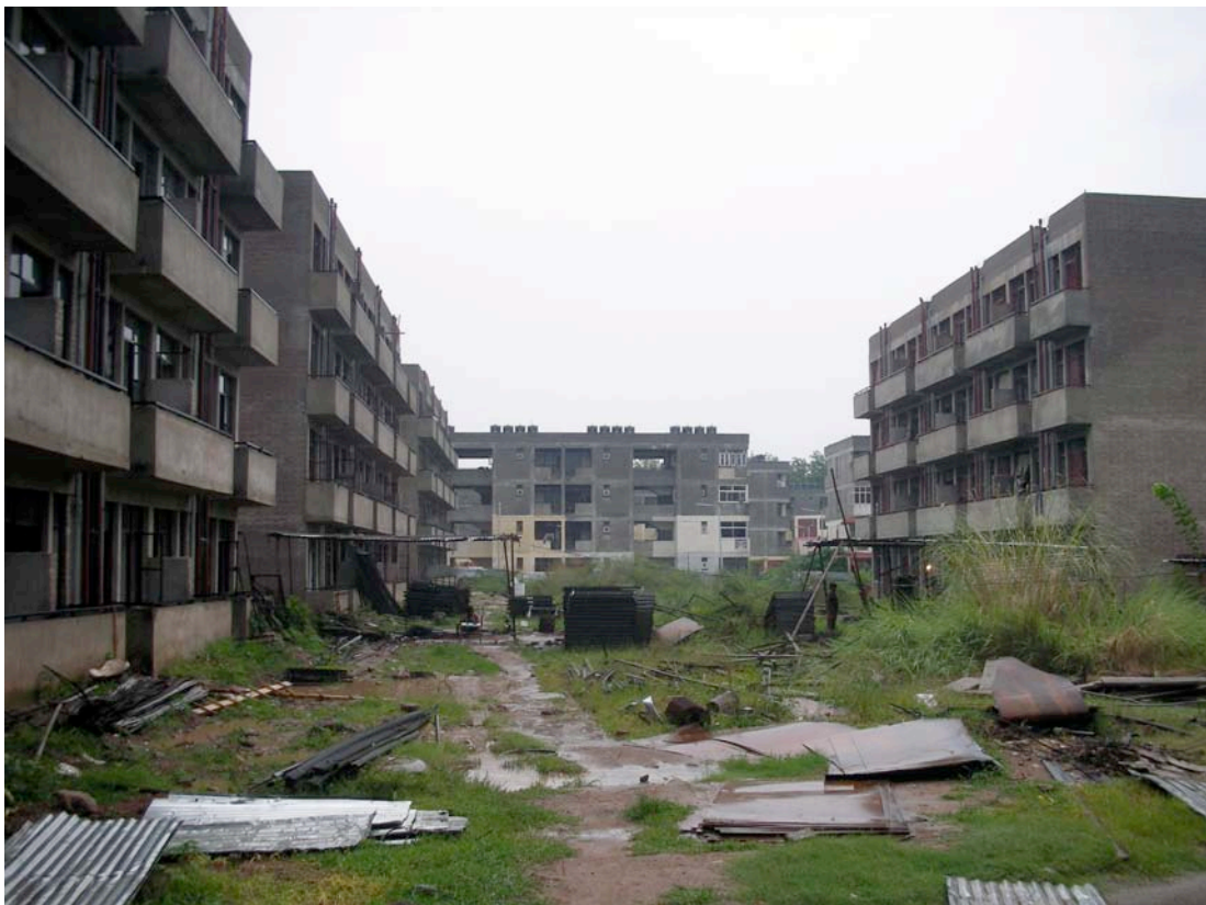
The Dadu Majra Rehabilitation Colony, 2011
